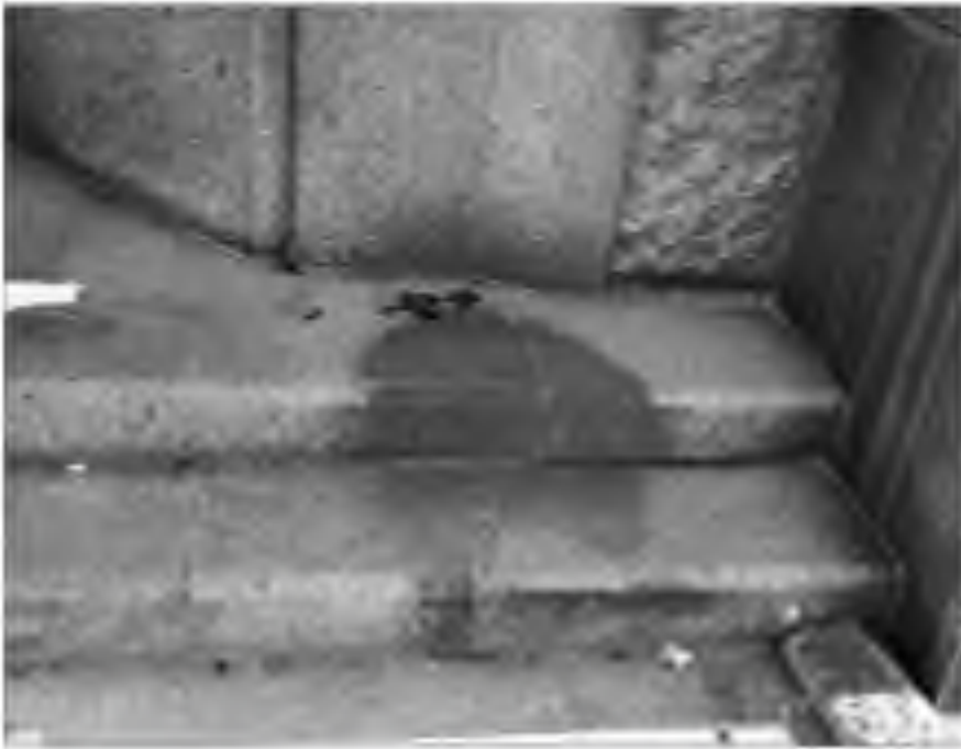
Figure 3.7 Shadow effect: Unidentified photographer, flash burns on steps of Sumimoto Bank Company, Hiroshima branch. (Courtesy of National Archives and Records Administration, Washington, D.C., photo no. 243-H-982.)
